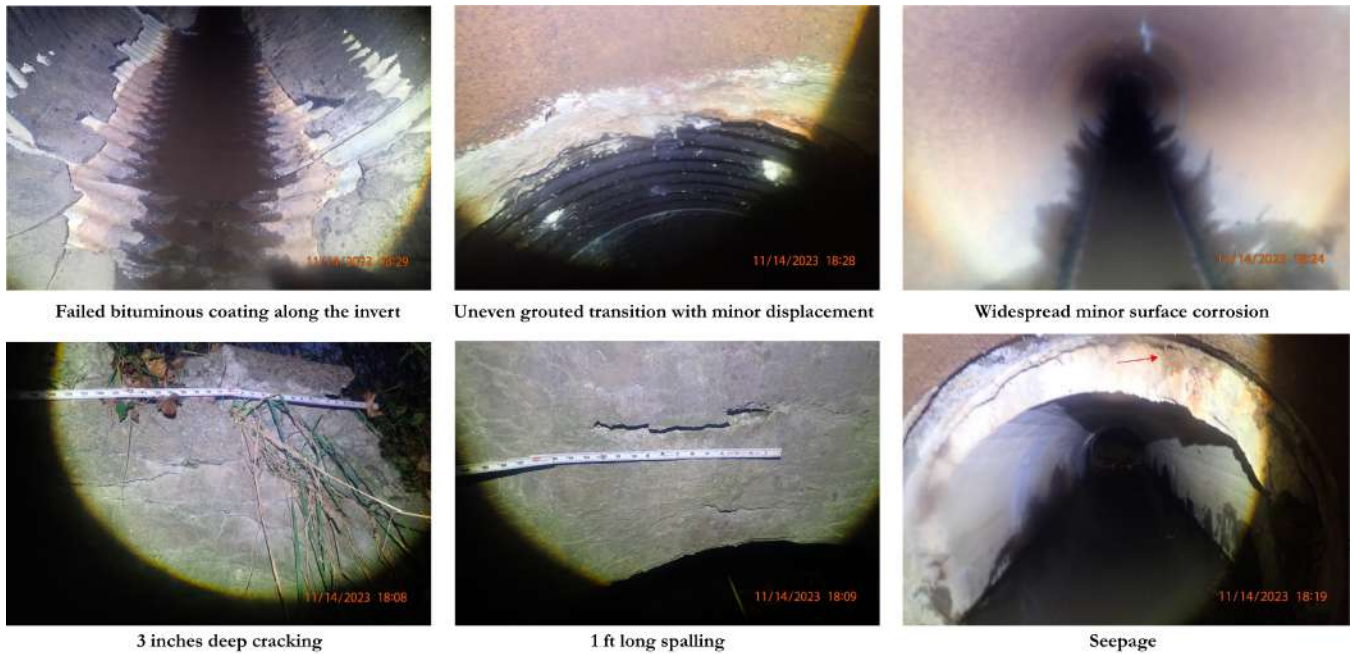
Fig. 4: Structure Inspection Report completed by NYCC on 11/14/2023 at Culvert - 110 (Royalton). The inspection was carried out manually by the inspector using hand tools, including a digital camera, folding ruler, hammer, and tape rule. The report illustrates various degradation landmarks inside the culvert.
